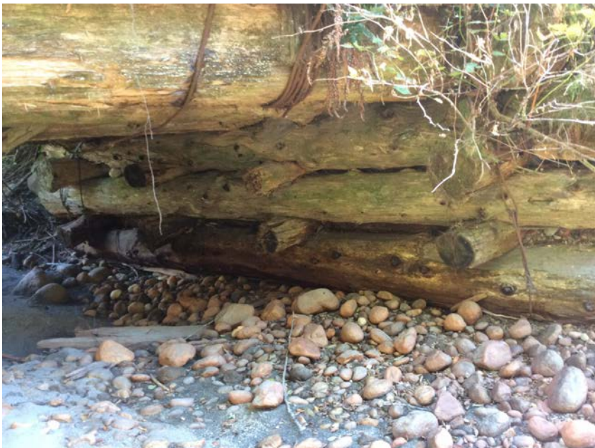
Left Bank Abutment when facing downstream
