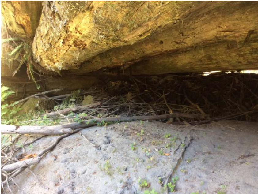
Right Bank Abutment when facing downstream
