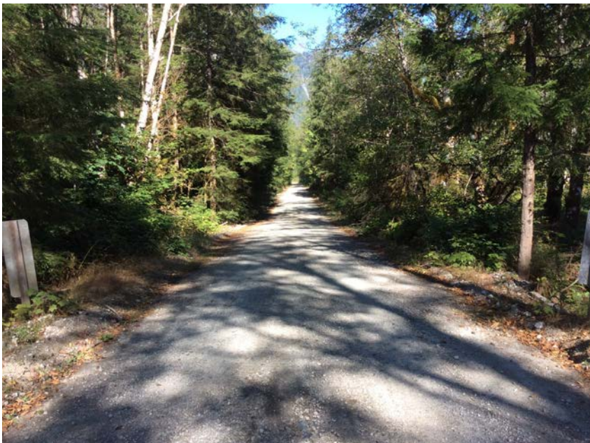
Right approach viewed from bridge
