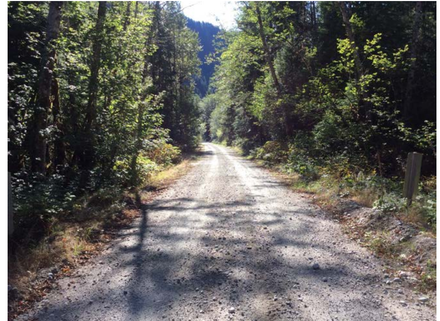
Left approach viewed from bridge
